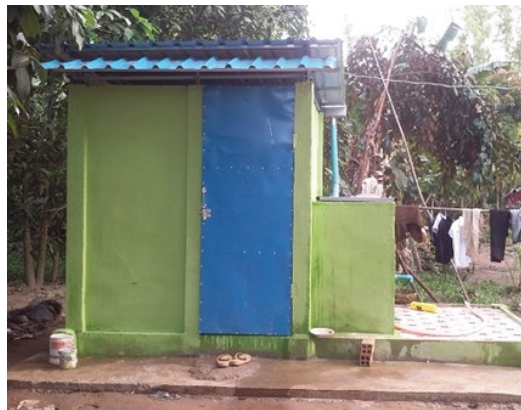
2. Latrine built by LOLC WASH loan
