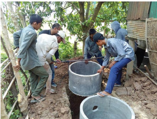
1. Water sanitation project in construction from LOLC WASH loan
